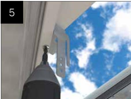
NOTE: The transom bracket CHA001 MUST be trimmed and adapted to suit situations where a transom bar, valley and insulated internal pelmet vertical frame intercept, as shown above.
