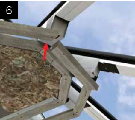
Using drywall screws, attach battens into steel bolsters/stub steel bolsters.
