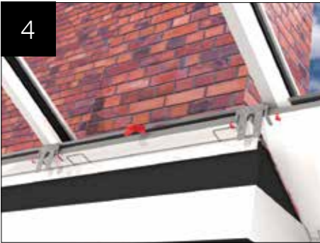
Fit the polycarbonate modesty panels and bend over bracket legs to secure.
