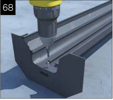
Screw the flashing trim to the ridge top cap through the screw port. Use a 4.2mm x 13mm self drilling screw (not supplied).
