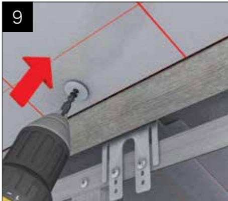
Fasten through the board and into the glazing bars using the drywall screw provided (3.5 x 50mm) and with a washer (kit of 25) behind the head to offer additional support to the board. Use location plan to identify board positions. Use tape LVFT045 - foil sealing tape - tape ALL joints of 25mm insulation.
