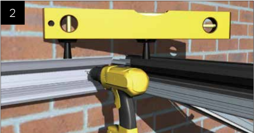
Assemble as much of the main Georgian (or vic) roof side of the 'P' shape as possible. CHECK THE PITCH. Ensure the full ridge is level. Separate the two part half ridge. REMOVE THE RAIN BAFFLE UPPER LEG. Fit the back section of the half ridge in position, level across the PVCu top carriages (as shown), then secure to the host wall with anchor bolts suitable for the substrate. The first anchor to be 50mm away from full ridge, the second 250mm and then at max 600mm centres.
