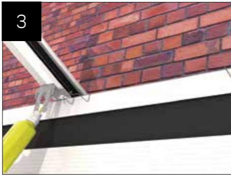
If the area around the box gutter is glazed fit brackets in marked positions on the bars as per standard installation.
