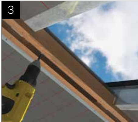
IMPORTANT: POSITION CLOAKING PANEL ASSEMBLY INLINE WITH THE CROSS BATTEN (AS SHOWN) SCREW FIT INTO POSITION.
