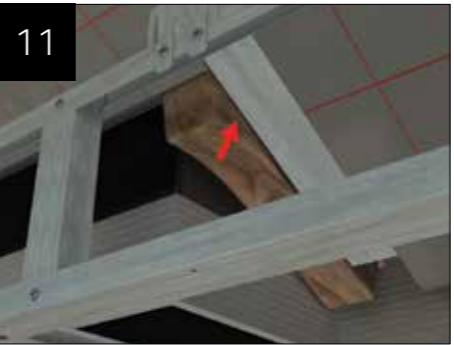
In the case of an L-shaped conservatory, where the box gutter returns around the house wall If the distance between the side gutter fascia and the adjacent transom bar is less than 100mm, 90mm insulation will not be specified and a gap will remain- in this case, insert mineral wool to fill the cavity.
