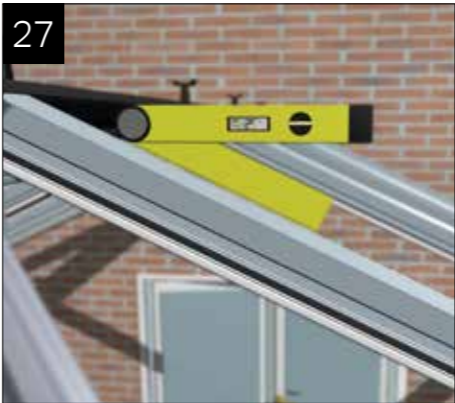
Check that the pitch of the roof is correct. Your Surveyor should have provided a drawing/a copy of the roof confirmation which displays the pitch.
