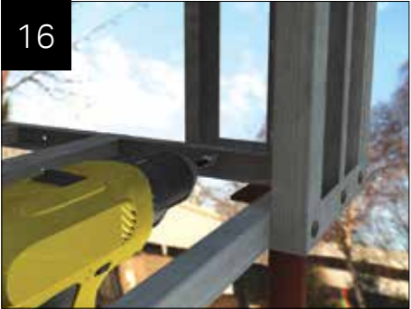
Fit the valley corner infill panel to the horizontal frame, level up and secure to the valley plate.
