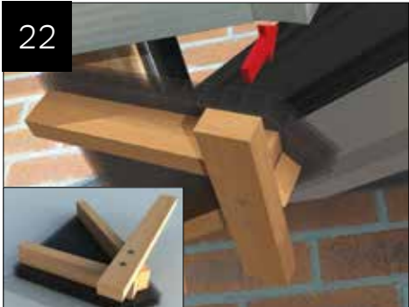
Offer up the cassette assembly into position.
