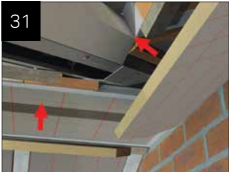
Fit 25mm insulation.
