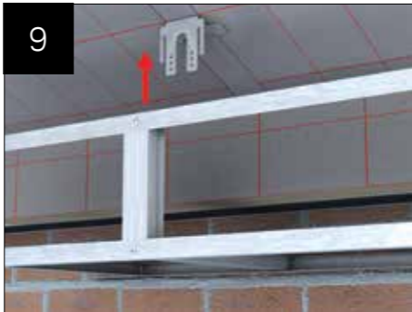
Offer up into position and fit in place using CHAA006 (bag of 25).
