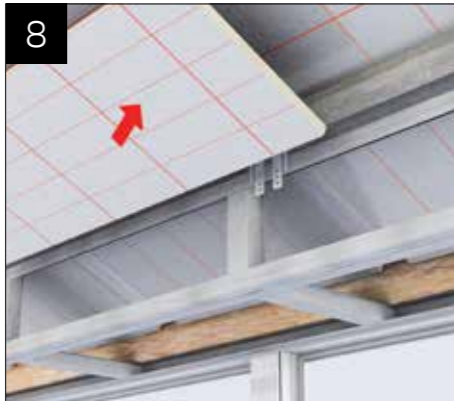
Next fit the 25mm insulation board, which is 590 x 2400mm. These boards must be laid at right angles to the glazing bars and run across the bars.
