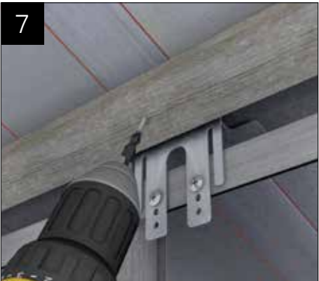
At eaves attach batten into steel bolsters using dry wall screws.
