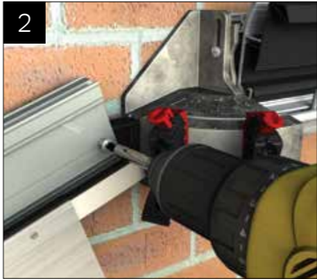
Prior to attaching the starter bar to the mounted starter bar bracket, remove the M6 taptite screw. Locate the bar on to the bracket and on to the single bolt placed in the eaves beam, re-insert the screw.
