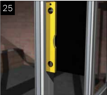
Ensure the window frames are plumb.
