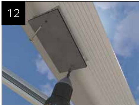
Fit valley plate, with foam backing towards the valley, to the valley wing central connector using CHA017 (2 X 4.8 X 70mm self tapping screws).
