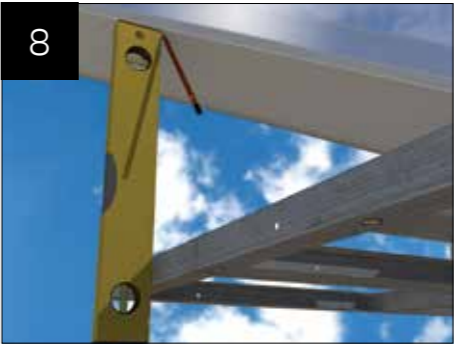
Using a level, plumb up off the horizontal frame and mark the outer bottom edge of the valley cladding on both sides (Mark "A").
