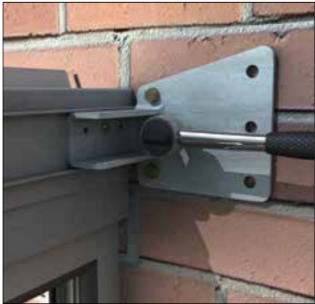
SUPER DUTY EAVES BRACKET: Where the Super Duty Eaves beam has been specified, bracket SEWC002 (left and right handed) will be supplied. This should be fitted to the eaves beam using X3 M5 X 12 tapite screws (supplied). This should then be fitted to the host wall using a minimum of 4 fixings suitable for the substrate (not supplied).
