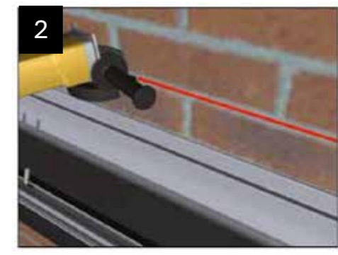
Whilst still supported, pull gutter away from the wall for access and grind a channel in the masonry for flashing. Blow out any dust in the channel.
