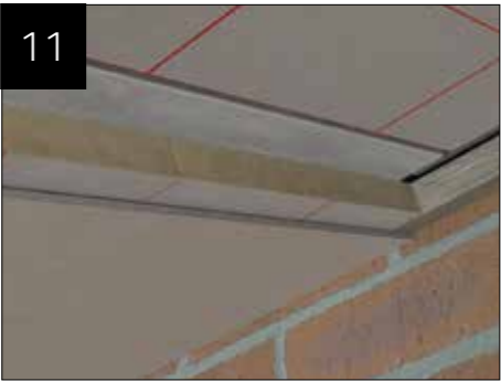
When fitted, the 25mm insulation should butt up to the batten, and the plasterboard should fix through into the underside of the batten as shown.
