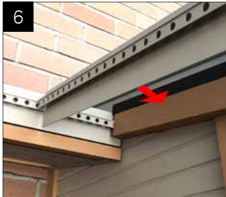
Fit LVCT trim - ensure it touches glass. Screw fit.
