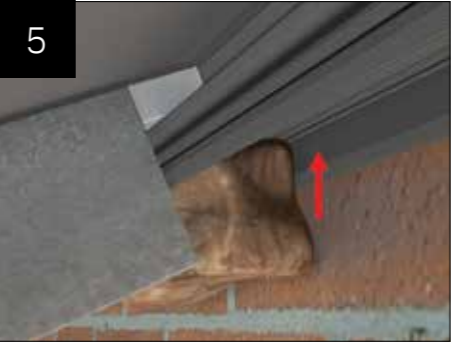
Insert mineral wool along the length of the wallplate.
