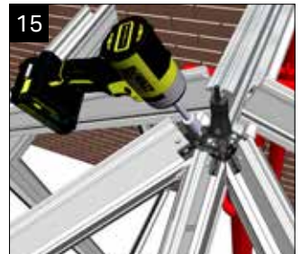
Once level and pitches are correct, tighten fixing in the Spider arms using a 8mm socket bit. This locks the position of the arms.
