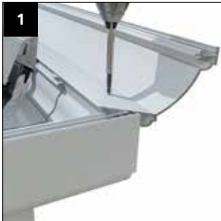
1 Temporarily support and fit the upper Cornice section, using the fixings provided (FSD-42-19).
