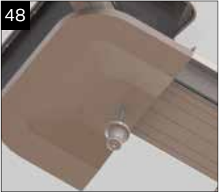
Offer up the internal radius end cap, use the threaded bar and the retaining boss to secure the internal cap in position. The threaded bar may require cutting to suit.
