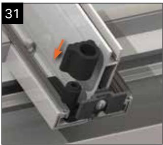
Snap off a gromet from the kit, this will slot over the upstand on the glazing stop. Repeat spets 35 & 36 for all glazing bars on the roof.
