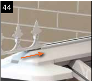
If cresting is specified, insert the cresting down the channel on the ridge top cap. This may require trimming to suit.
