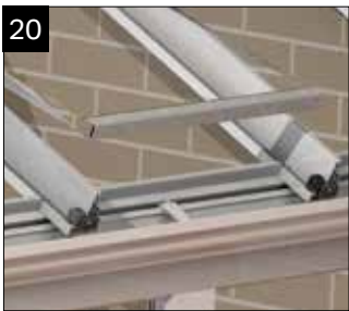
20 At this point the roof should be glazed. Any ridge support may be removed. Insert the glazing between the rafters ensuring that it is centralised.
