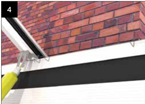
4 Fit brackets in marked positions on the bars as per standard installation
