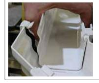
Squeeze gutter together when fitting to avoid the gasket being dragged out of position.
