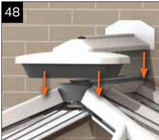
Fit the ridge top cap complete with flashing trim and crown cap to the ridge.
