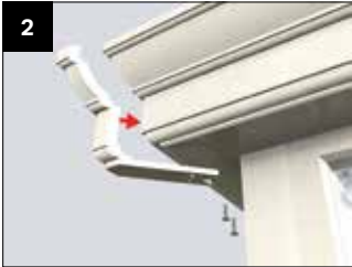
Whilst ensuring that the corner remains located in position, screw fix using self drilling screws CRN007
