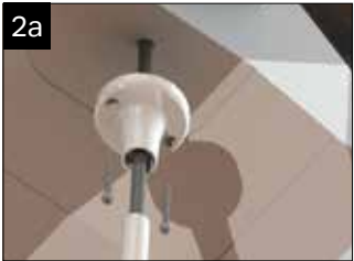
Offer up the internal radius end cap, retain this using the tie bar ridge fixing cover and two self tapping screws provided. Cut the PVCu conduit to suit.
