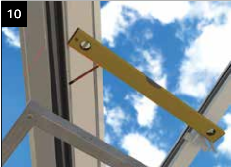
Using the bracket positions, level through and mark off the valley marked 'C'.
