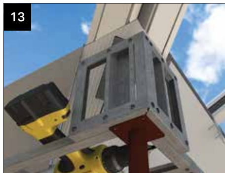
Valley infill panel fitted to horizontal frame, as image 10.
