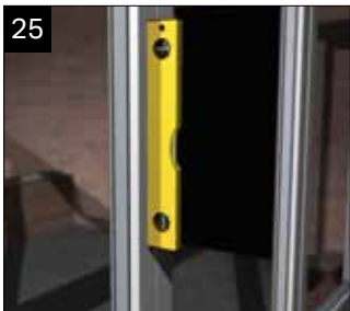
Check the window frames are plumb.
