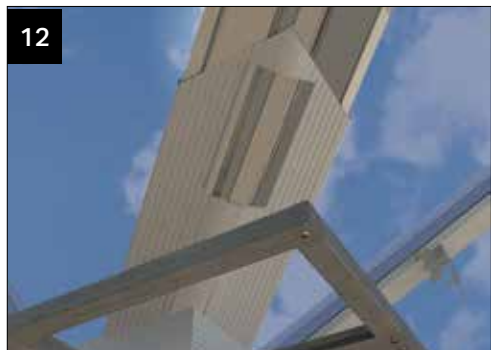
Fit the valley plate CHA016 (refer to steps 1-5, valley standard classic).
