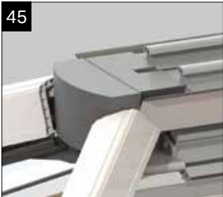
Take the semicircular foam piece and insert it into the front of the crown point. This may require sculpting to suit the situation.
