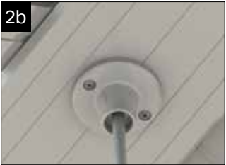
Thread the tie bar rod into the ridge fixing cover. Measure the drop of the rod and cut to suit the position or the tie bar boss ring.
