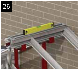
Ensure the ridge is level.
