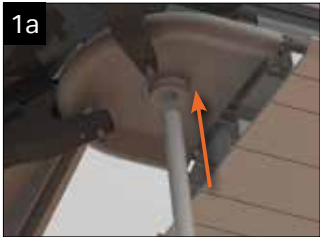
Tie bar at finial Insert the tie steel rod thread into the base of the spider. Measure the drop of the rod and cut to suit the position or the tie bar boss ring.
