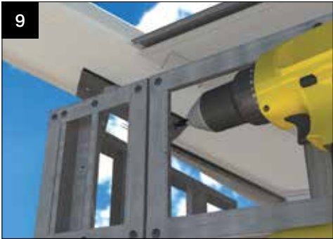
Fit the vertical frames. Fix the frames into the valley corner infill and the horizontal frames.
