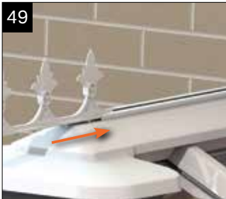
If cresting is specified, insert the cresting down the channel on the ridge top cap. This may require trimming to suit.
