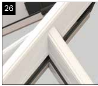
26 When fitting the jack rafter top caps, seal where the cap meets the hip top cap. The jack rafter top cap should sit tightly against the hip cap.
