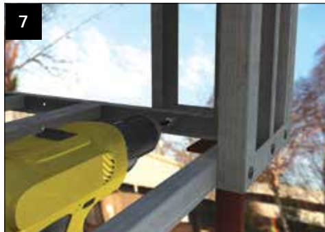
7 Fit the valley corner infill panel to the horizontal frame, level up and secure to the valley plate.
