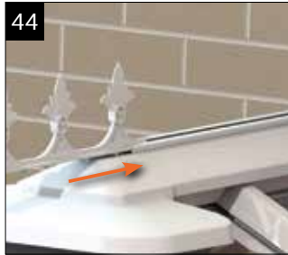
44 If cresting is specified, insert the cresting down the channel on the ridge top cap. This may require trimming to suit.
