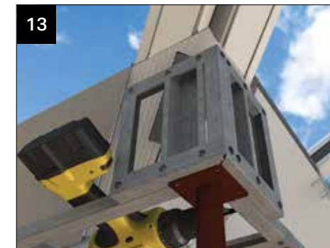
13 Valley infill panel fitted to horizontal frame, as image 10.
