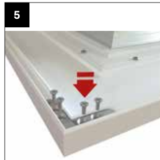
5 Secure each corner using the cleats (CRN001) and fixings provided (CRN006). The gutter and glazing should now be fitted (see main guide). Check integrity of all gutter joints before proceeding further.
