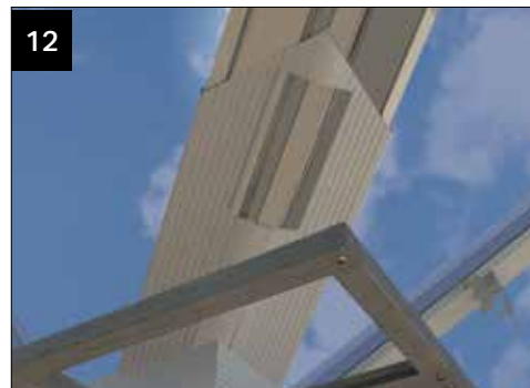
12 Fit the valley plate CHA016 (refer to steps 1-5, valley standard classic).
