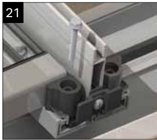
21 Ensure the glazing stop is pressed tightly up against the end profile. When in position use the fixings provided to fix the glazing stop down into the bar as shown. Ensure clip offers maximum support to glazing at all times.
