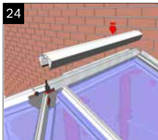
24 Fit ridge capping by locating barbs in ridge profile and knocking down along its length. Use a timber drift and dead-blow hammer to avoid damaging the capping.
