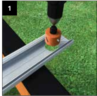
1 Decide the position of the gutter outlet. Using a 68mm dia hole saw, cut the hole for the down pipe in the lower section.
