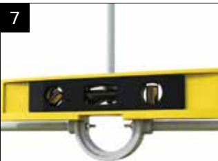
Now, finally check that the horizontal elements are level and the vertical element is plumb. CHECK THAT THE SIDE FRAMES ARE STILL PLUMB. Spanner tighten the boss nyloc nuts.
