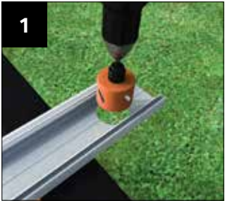
Decide the position of the gutter outlet. Using a 68mm dia hole saw, cut the hole for the down pipe in the lower section.
