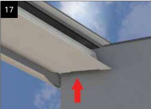
Valley cladding being fitted against pelmet . After plasterboard and skim.
