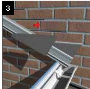
Place Conservaflash into the ground out mortar joint at the gutter end, ensuring lower edge locates into the 'J' soaker.
