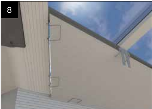
Attach the cloaking panels and fit as shown in the main pelmet installation guide. (page 16).
