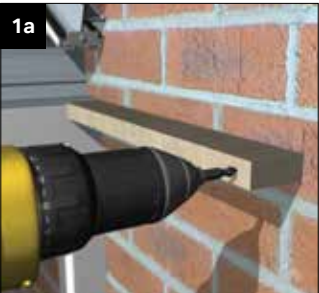
GUTTER RETURN DETAIL - If the gutter returns along the host wall (shown above) complete steps 1A and 1B after step 4 of the general installation. Ensure the treated timber baton (49mm x 20mm) is level, then fix into position.
