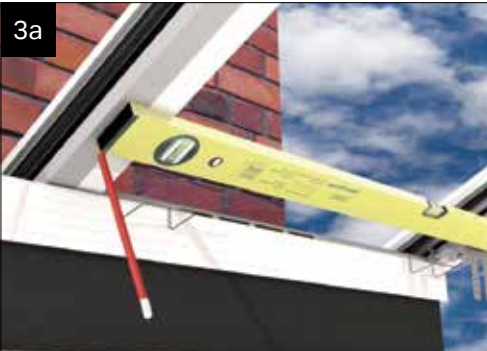
FITTER TIP: If possible, check and line through with the bracket position on the adjacent full length bar. Mark the bracket positions on the bars off the box gutter.
