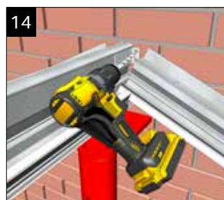
Drill through the holes in the fixing bracket and fix back using an appropriate masonry anchor. Fix frames.
