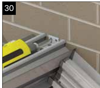
Drill through the holes on the ridge fixing bracket and secure with the correct masonry anchor. Now fasten the frames to the host wall and the dwarf wall.
