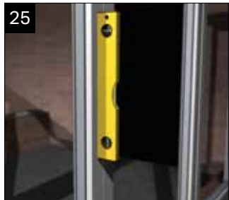
Check the window frames are plumb.
