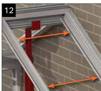
Check that the starter rafter and the first rafters are parallel. Ensure all bolts at both eaves and ridge are fully tightened.
