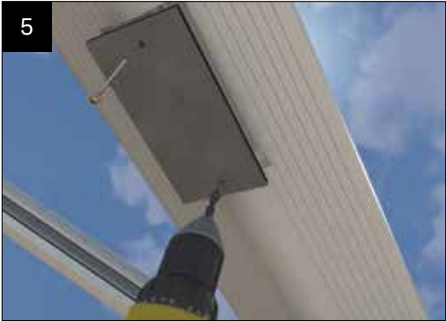
Fit valley plate as shown to the valley wing central connector using CHA017 (2x4.8x70 self tapping screws).
