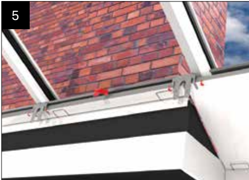
Fit the polycarbonate modesty panels and bend over bracket legs to secure.
