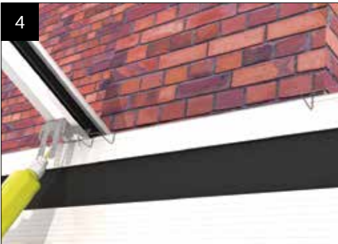
Fit brackets in marked positions on the bars as per standard installation and fit closure trims CHA---GR/5 according to layout plan.
