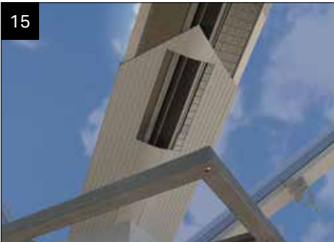
Fit the valley plate CHA016 (refer to steps 1-5, valley standard)
