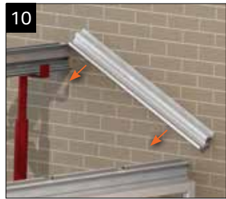
Continue to support the ridge and offer up the starter bars at the host wall. Locate on to the single bolts at the ridge and eaves.
