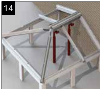
Using the location plan, repeat these steps until all rafters that meet the ridge have been fitted in the correct position and have been secured.
