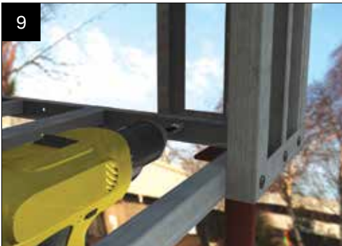
Fit the valley corner infill panel to the horizontal frame, level up and secure to the valley plate.
