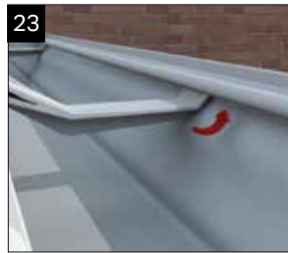
Clip the front of the bracket into the lip on the gutter. PVCu components like the gutter are easier to manipulate when warm. In cold conditions more 'force' may be required.
