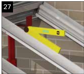
Check that the pitch of the roof is correct. Your Surveyor should have provided a drawing/a copy of the roof confirmation which displays the pitch.
