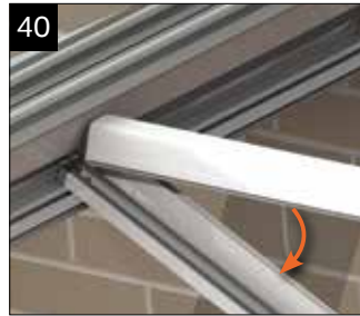
Once the roof has been fully glazed and glazing stops secured, work your way around the roof fitting the glazing bar top caps. These should be angled in at the ridge first before forcing the top cap down along the bar length. Ensure to fully engage w grip clip.
