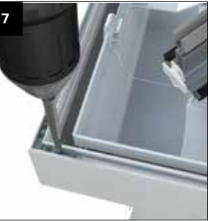
As shown in step 5 it may be advisable to temporarily support the Cornice whilst fixing. Secure corners using the cleats (CRN001) and fixings provided (CRN006).
