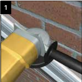
At this stage it is easiest to mark and cut out for the lead flashing. For best results always grind a 35mm deep slot to allow Conservaflash to be let into the wall. Brush out any dust from the channel.
