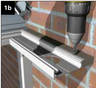
Secure lower section using fixings provided (CRN007)
