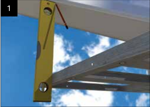
Using a level, plumb up off the horizontal frame and mark the outer bottom edge of the valley cladding on both sides (Mark 'A')
