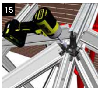
Once level and pitches are correct, tighten fixing in the Spider arms using a 8mm socket bit. This locks the position of the arms.
