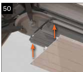
Moving inside the roof, fit the ridge undercladding to the ridge.
