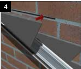
The unique integral mechanical retention wedge clips bite into the brickwork ensuring positive location. Insert the next stepped flashing (using sealant on the back), ensuring it overlaps to marked minimum. Continue up the roof, both slopes, with stepped flashings.
