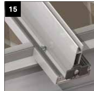
Attach all the rafter using the location plan provided to check each bar's final position with its corresponding label.
