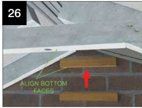
Fit a length of timber batten to the host wall, ensuring that its underside lines through with the underside of the struts (LVTS001/LVTS002). This will provide a fixing point for the ridge board fitted in the next step.
