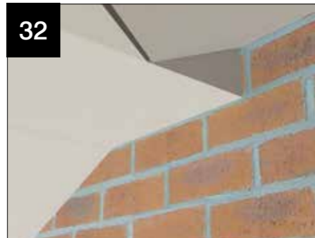
Now fit the plasterboard – the detail where the valley abuts the host wall should look as shown. Fitters tip: fit the small triangular segment of plasterboard shown first, allowing space for the upper adjacent board to slide in above it, as there will be nothing to screw to at this point.
