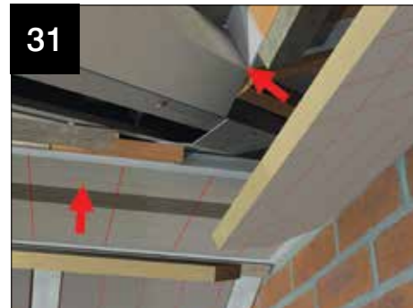
Fit 25mm insulation.
