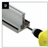
Attach the glazing rafter end cap brackets - as access restriction may prevent easy fixing later. These are not required on hip rafters.
