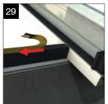
Peel back a small tab of the protective film on the glazing support from the eaves.
