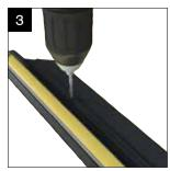
Drill the eaves beam at 100mm from each end and drill a minimum of 4 holes at a Max of 400mm centres using appropriate clearance drill. Now take the eaves beam and ensure correct number of bolts are slotted into eaves beam.
