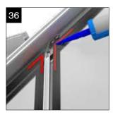
If the lantern has jack rafters. At the corners of the glazing that meet the jack rafter bracket, apply MS polymer to the surface of the glazing as shown above to create a order is, hip top caps followed by jack barrier. This should be positioned towards the edge of the glazing as to be obscured by the top caps once they are installed.
