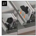
Snap off appropriate handed glazing stop. Place this onto the base of the glazing rafter. Snap off a grommet from the kit, this will slot over the up-stand on the glazing stop. Repeat this for all glazing rafters on the roof, excluding hip rafters as these will be fit with classLOCKs.
