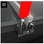
Push the glass stops up to meet the glass end profile, ensure that the lower edge of the glazing is running parallel to the kerb. Then using fixings provided secure the glass stops in place.
