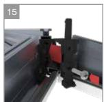
bracket over the left and right hand parts and bolt into the ridge. Repeat process at the opposite end of the ridge.
