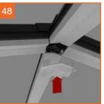
Clip the internal cover up into the ridgeLOCK from below. Ensure the clip feature meets the corresponding ridgeLOCK clip feature.
