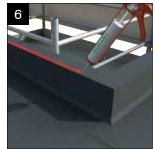
Apply a generous, continuous bead of sealant to the outer perimeter of the top surface of the kerb.
