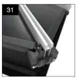
Ensure the glass units are pushed up towards the ridge and that the glazing is securely located behind the glassLOCKs at the hips.
