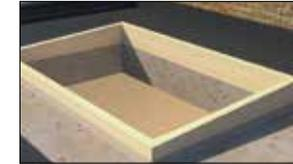
Construct the up stand to flat roof and fit roof covering.
