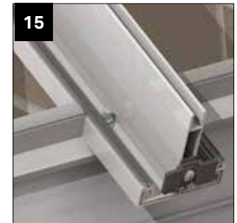
Attach all the rafter using the location pin provided to check each bars final position with its corresponding label.
