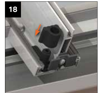
Snap off a gromet from the kit, this will slot over the upstand on the glazing stop. Repeat steps 17 & 18 for all rafter on the roof.
