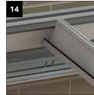
Ensure all the captivated bolts have been fitted, glazing pocket and ridge fascia. Offer up and secure the rafters on the bolts at the eaves and ridge. Secure with flanged M6 nuts.
