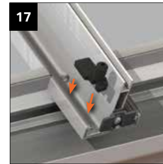
Snap off appropriate handed glazing stop. Place this into the base of the rafter.
